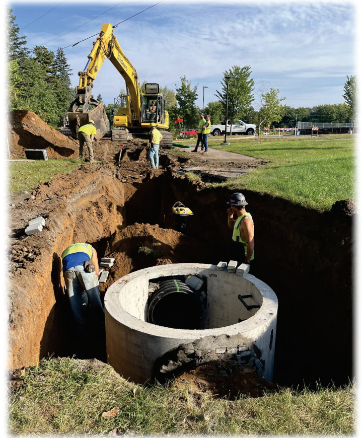
Storm Sewer Installation (2025)
