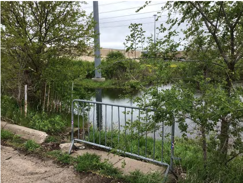
Image 2. Crumbling infrastructure and erosion along the existing parking lot creating safety hazards.
